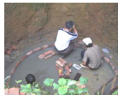
Construction of biogas units
